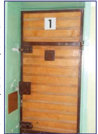
A typical cell door in an older facility.
