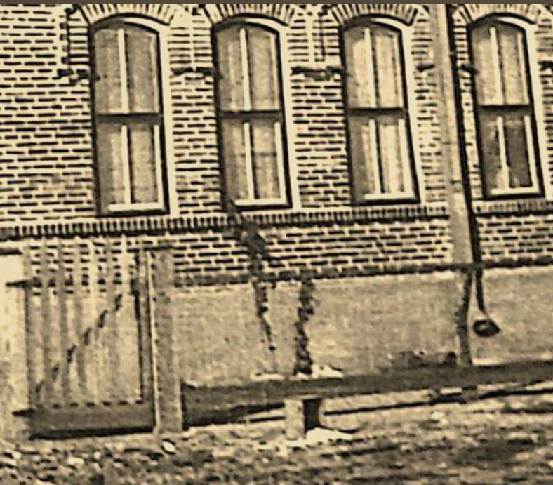
Atascosa County Jail- viewing Southeast, 1915
